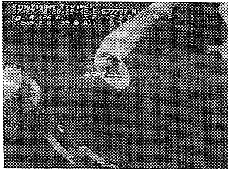
Figure 12 Dye Traces After Hot Stab Disconnection From Pipeline, Post Operation
